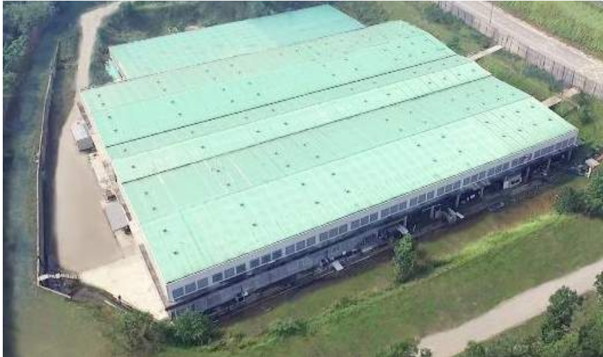
Below: Algaetech International's production site
